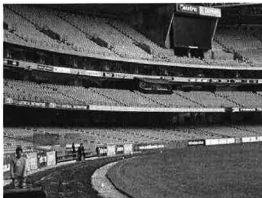
Figure 5.5 – Laying Artificial Turf Containing Recovered Rubber at Melbourne's Telstra Dome (April 2005)
