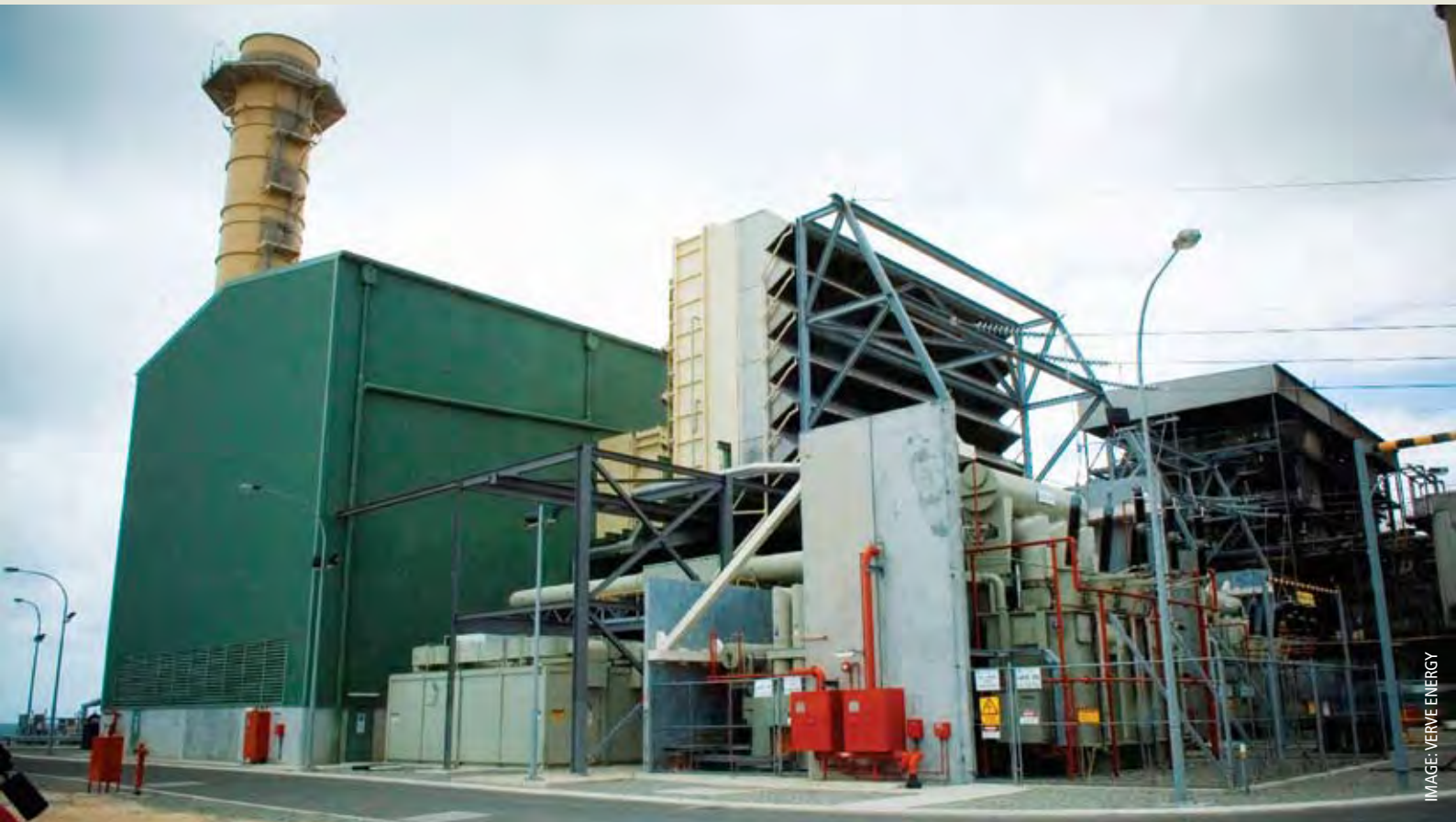
Verve Energy's gas-fired Cockburn Power Station.
