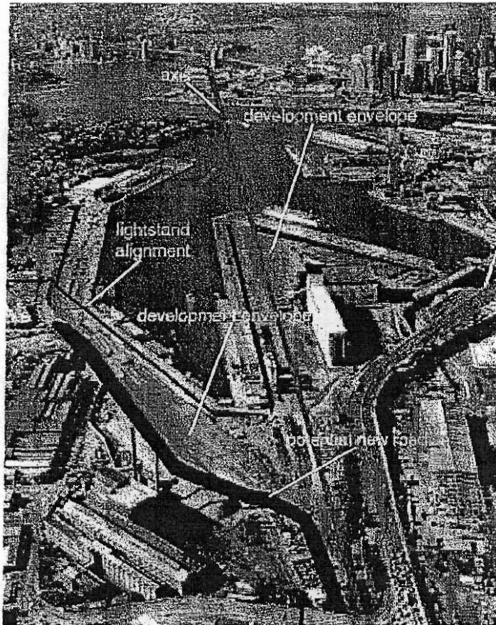
Fig 8. Alignment and location of any new structure should consider its broader context. Alignments exist in terms of existing infrastructure and relationships to the immediate surrounding environment. Note the axis line which parallels the White Bay shoreline and directly aligns with the main port entry (near Victoria Rd bridge) and the Port observation tower at Millers point. Other alignments can be used as reference points for the siting of buildings (such as a continuous setback to the wharf edge and the new road/rail corridor)
