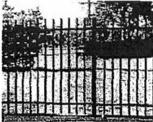
Fig 19. Proposed 1.2m high palisade fence
