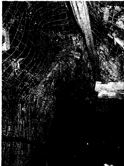
Figure 14: Install Face first pass roof - guttering
