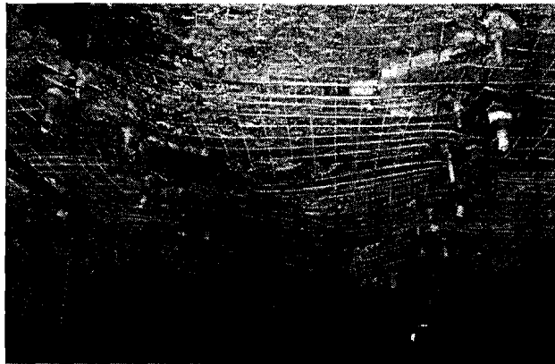
Figure 13: Install Face first pass roof – cable bolts
