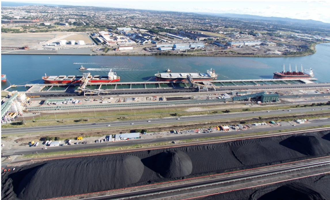
Figure 4: Shiploaders and berths at NCIG Terminal
