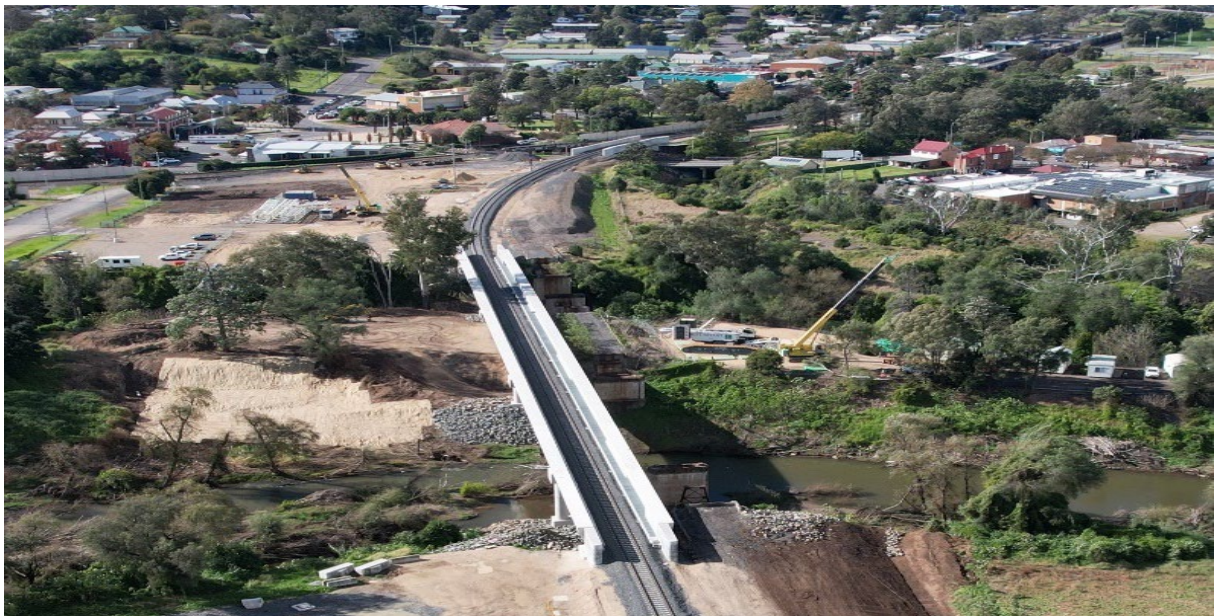
Figure 2: Completed Muscle Creek Hunter River Bridge and Bridge Street Bridge
