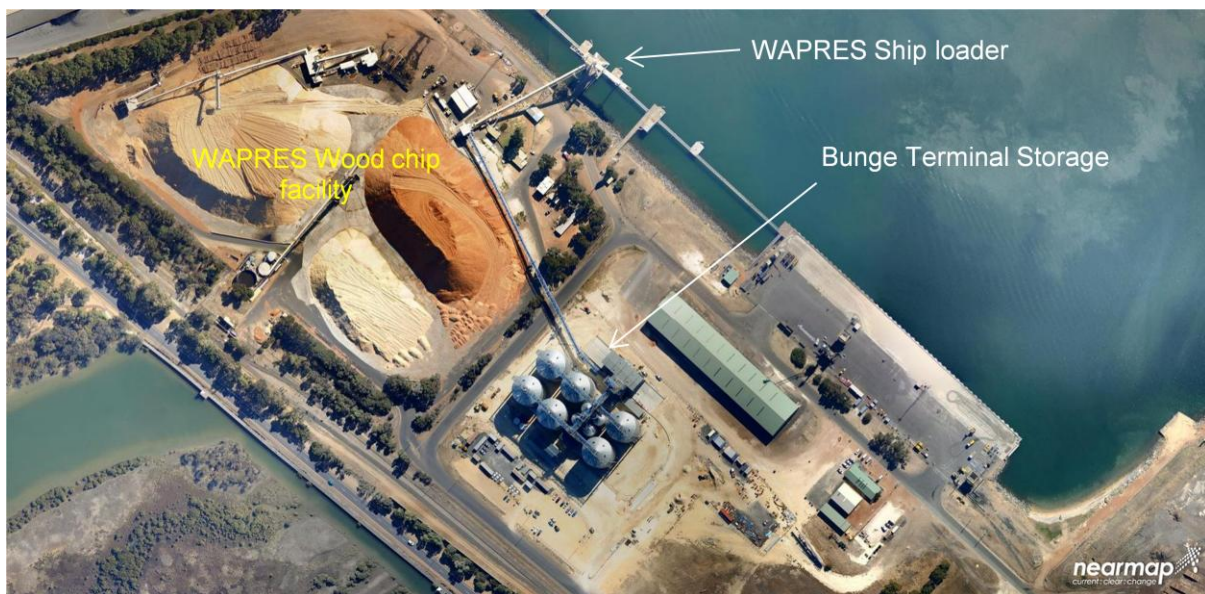
Figure 3 - WAPRES Facilities and Bunge Storage
