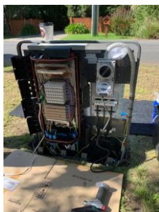
Figure D-3. An NBN micronode during installation (Credit: Tim Herring)
