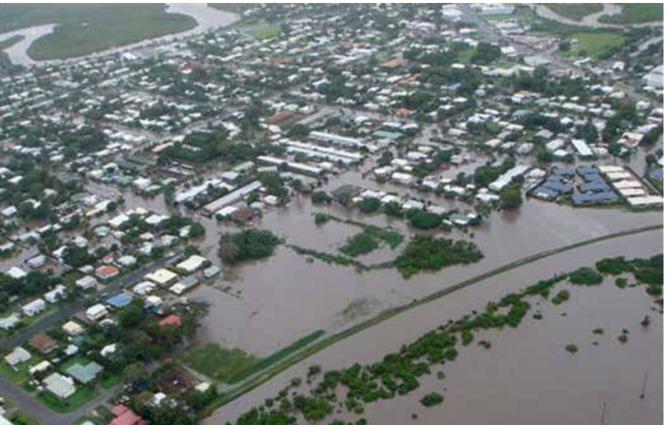
[Mackay during the February 2008 floods] Source: ABC news
