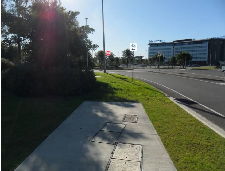
Above- A shared path on Lakeside Drive at Brisbane Airport which ends abruptly and does not connect to the road or another pathway. The path has remained this way for many years
