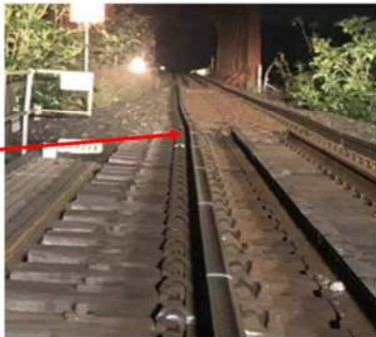
Figure 6: Muscle Creek Bridge abutment failure
