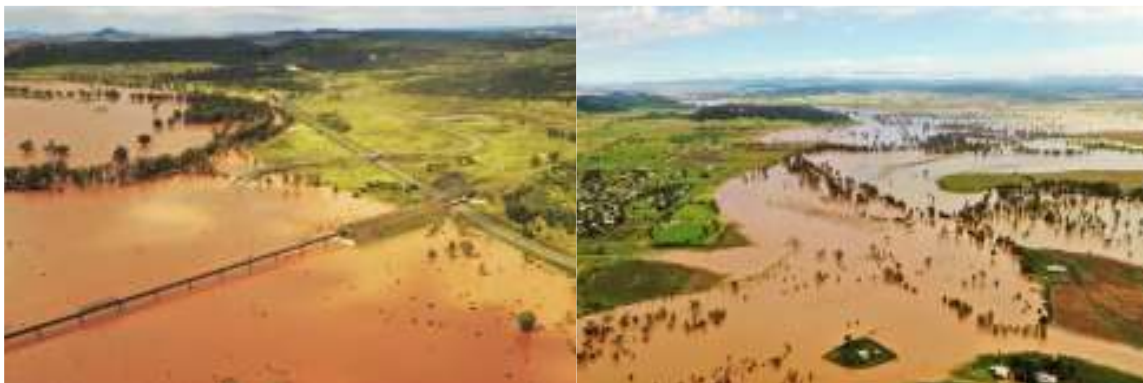
Figure 2 : Mine roads submerged in flood water just north of Boggabri 2
